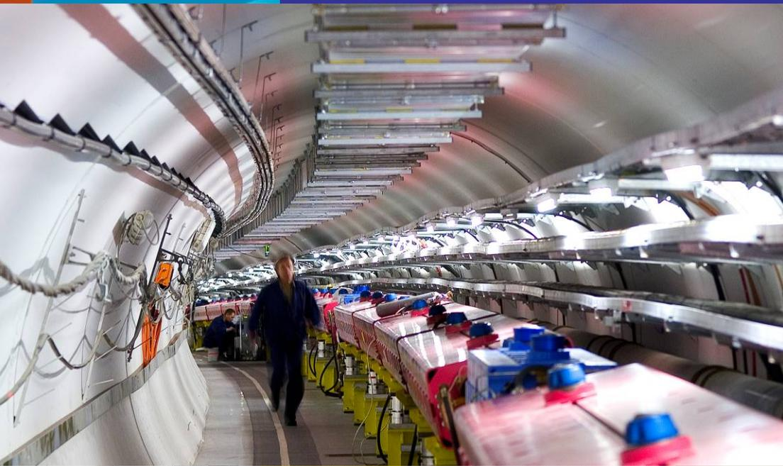
The protons beam line extracted from the SPS, and the target station
