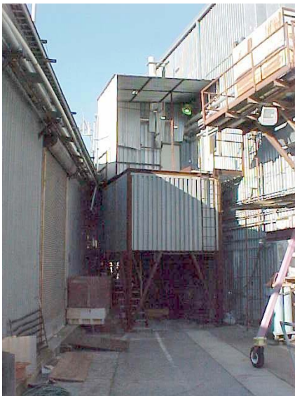
Two Story Structure Between Building 121 and Building 403
