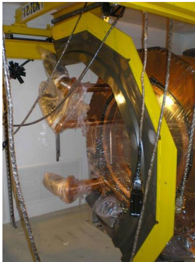
Pb arch installation
