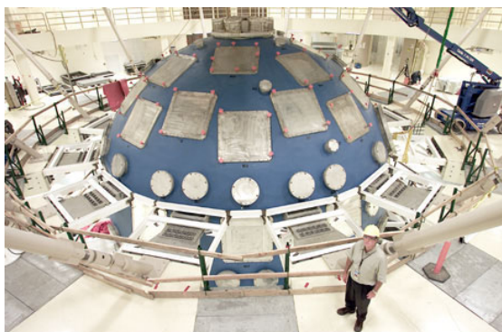
Target chamber with steel frameworks for catwalks being installed.
