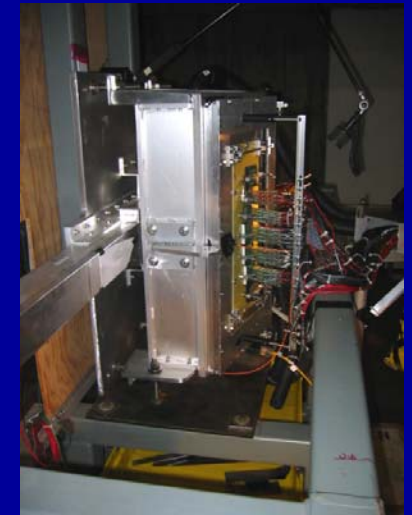
Electronics and cables
